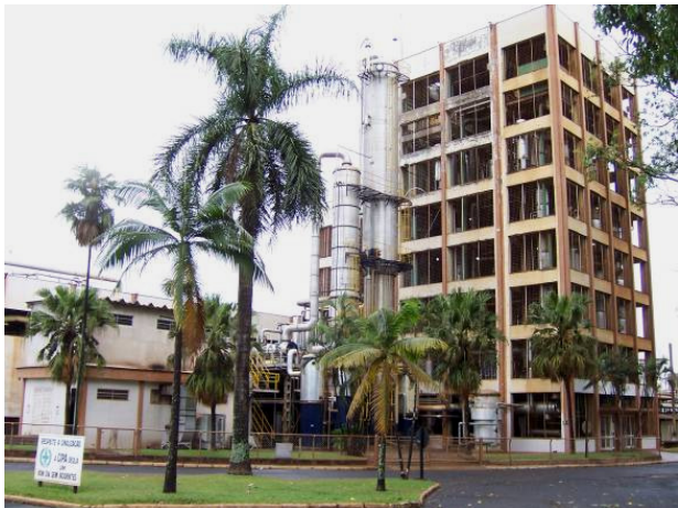
Sugarcane bioethanol plant (Brazil)
