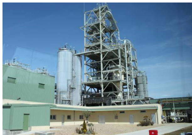
Lignocellulosic bioethanol plant (Spain)
